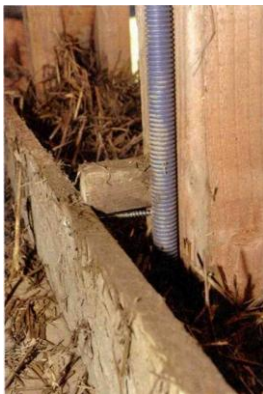
Fig.69: Le coffrage
